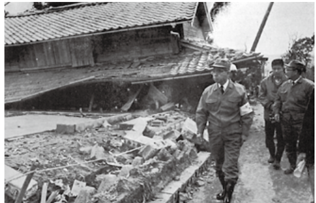
[Photo from Ebino jishin no kiroku ("A Record of the Ebino Earthquake"), published in 1969 by the Fire and Disaster Prevention Division, General Affairs Department, Miyazaki Prefectural Government]
