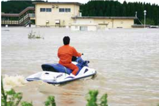
Oyodo River overflow (Miyazaki City)
